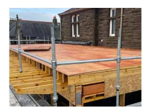
Work on the clubhouse is progressing very well. Almost all 'downtakings' have been completed, including the corner window at the existing Keg Store. As can be seen in the photograph, a full scaffold has been erected and the extension roof joinery works are proceeding at pace.
